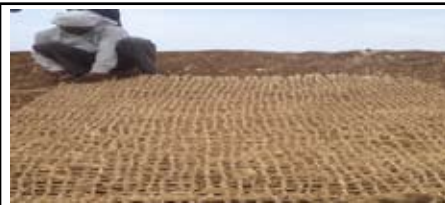
Fig.7: 8mm thick paddy straw Geomesh with 12x12 mm aperture size.
