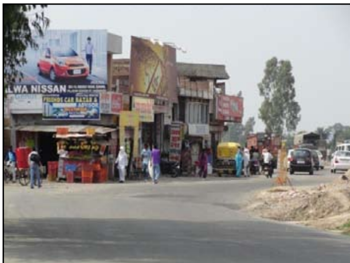
Fig. 5 : .At Km 143.500 LHS No lane marking, Poor Sight Distance
