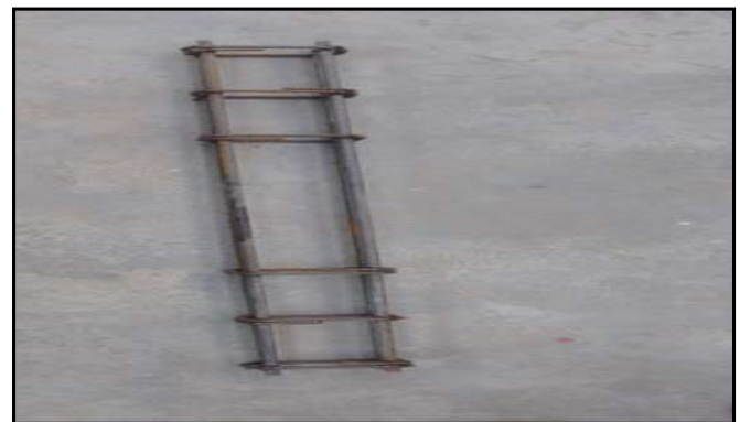
Fig 5 Cage of Beam
